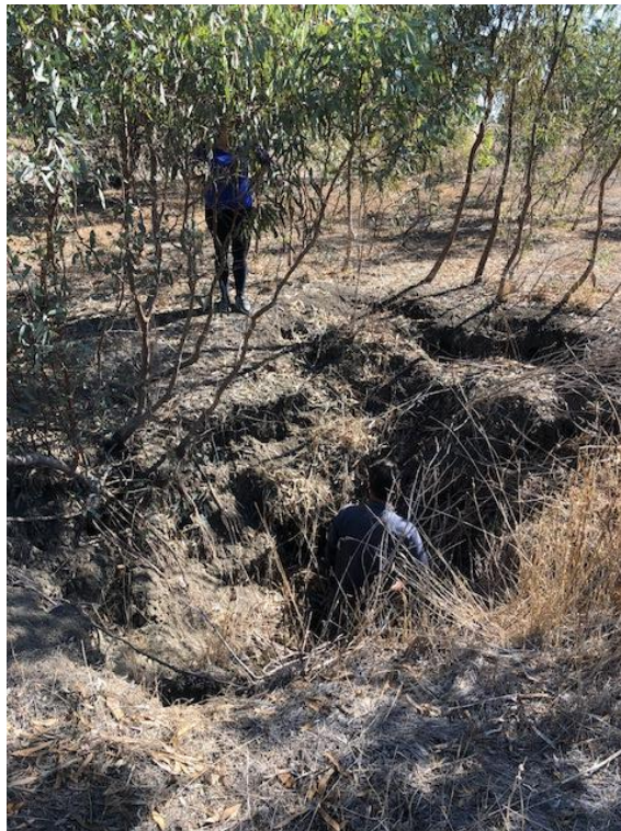
Runaway hole appearing at eastern end of Jamie Edwards property.
