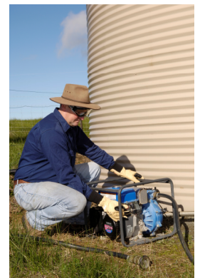
Regularly test pumps
