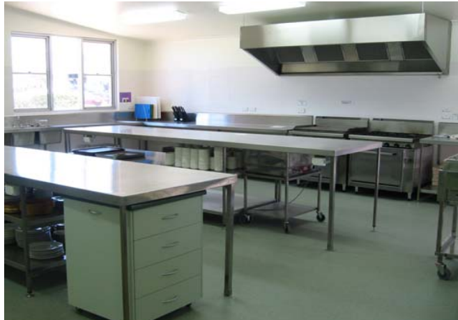
Bordertown Civic Centre – Kitchen Upgrade
