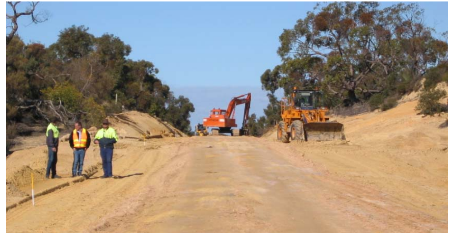
Work on the Hundred of Makin Road
